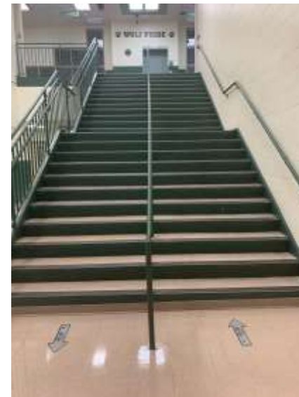
Bottom of Main Stairwell - Up on the Right, Down on the Right
